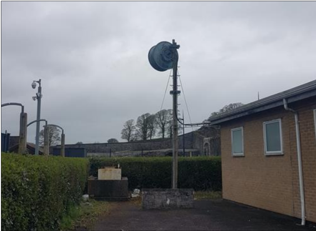
Figure 10. Telecoms Mast at Cashel
