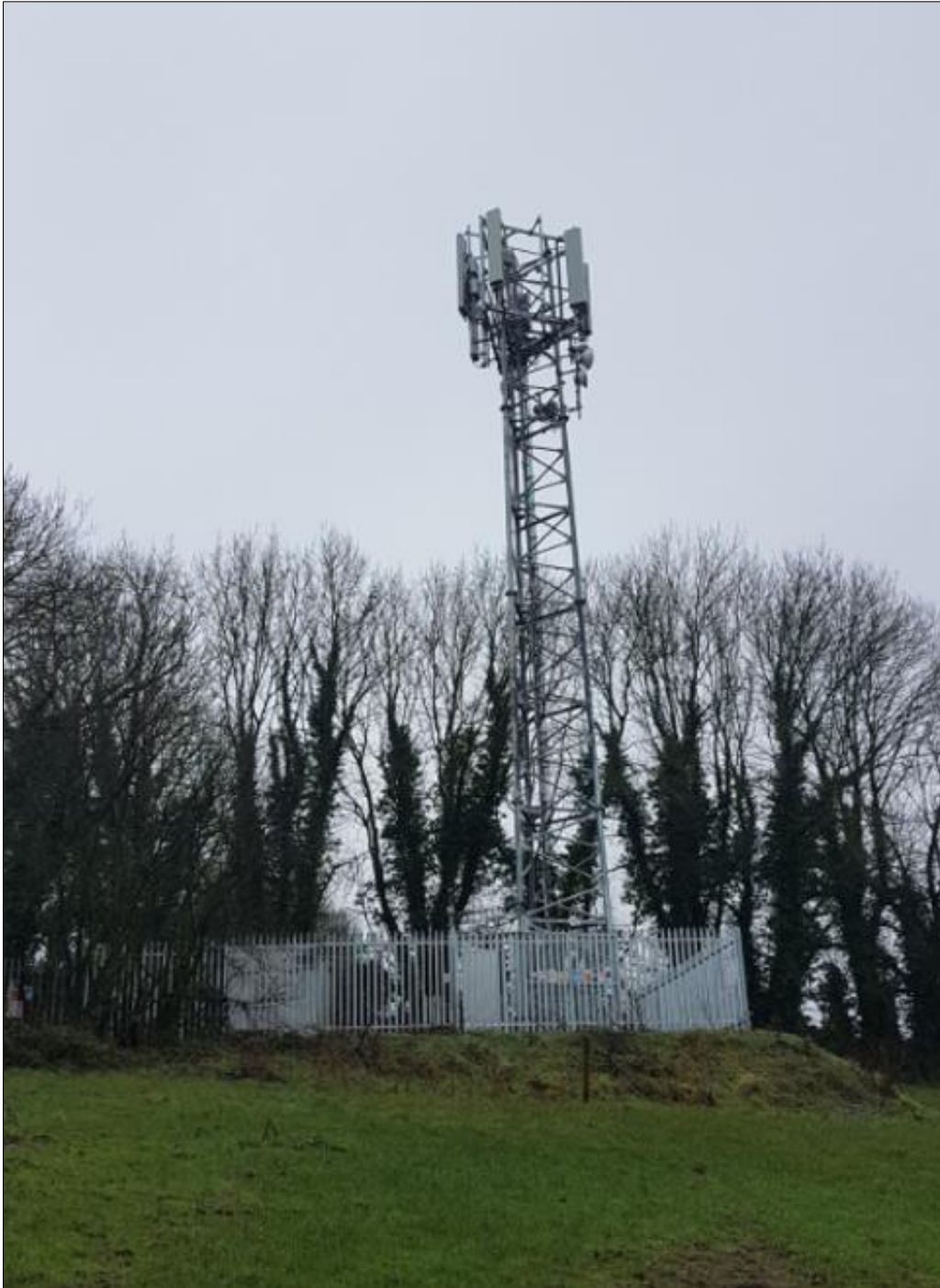
Figure 6. Telecoms Mast at Clonoulty
